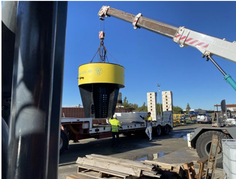
Large-scale 3200 X 3030 mm pump float for a 3-tonne 110kW pump
